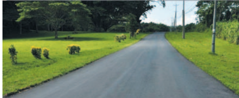
Repaving of Macqueripe Road
